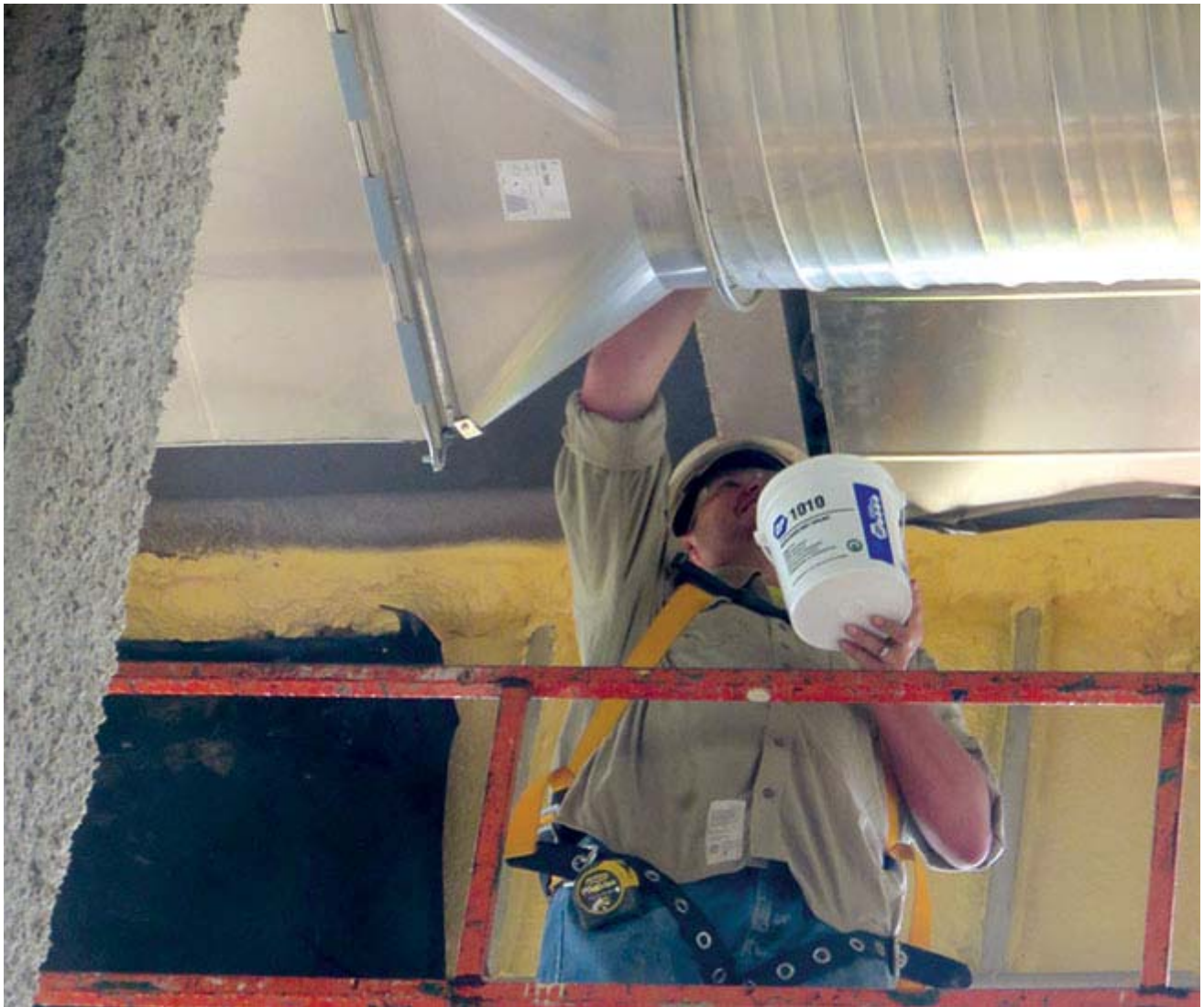
Vaughn Industries Mike Swirlain seals duct on a project in Columbus, Ohio.
